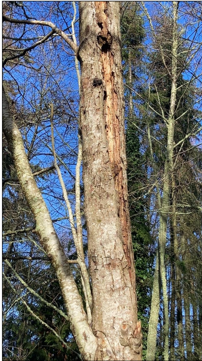
Photo 3: Tree 6603. Photo of decay.
